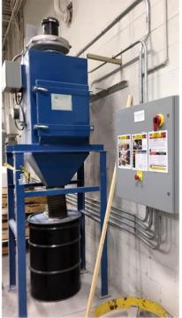
• 3Sigma provide a dust collector which is connected to the Contain-It™ chamber's dust port. The collector automatically starts and stops based on the status of the access chamber door (open or closed).
